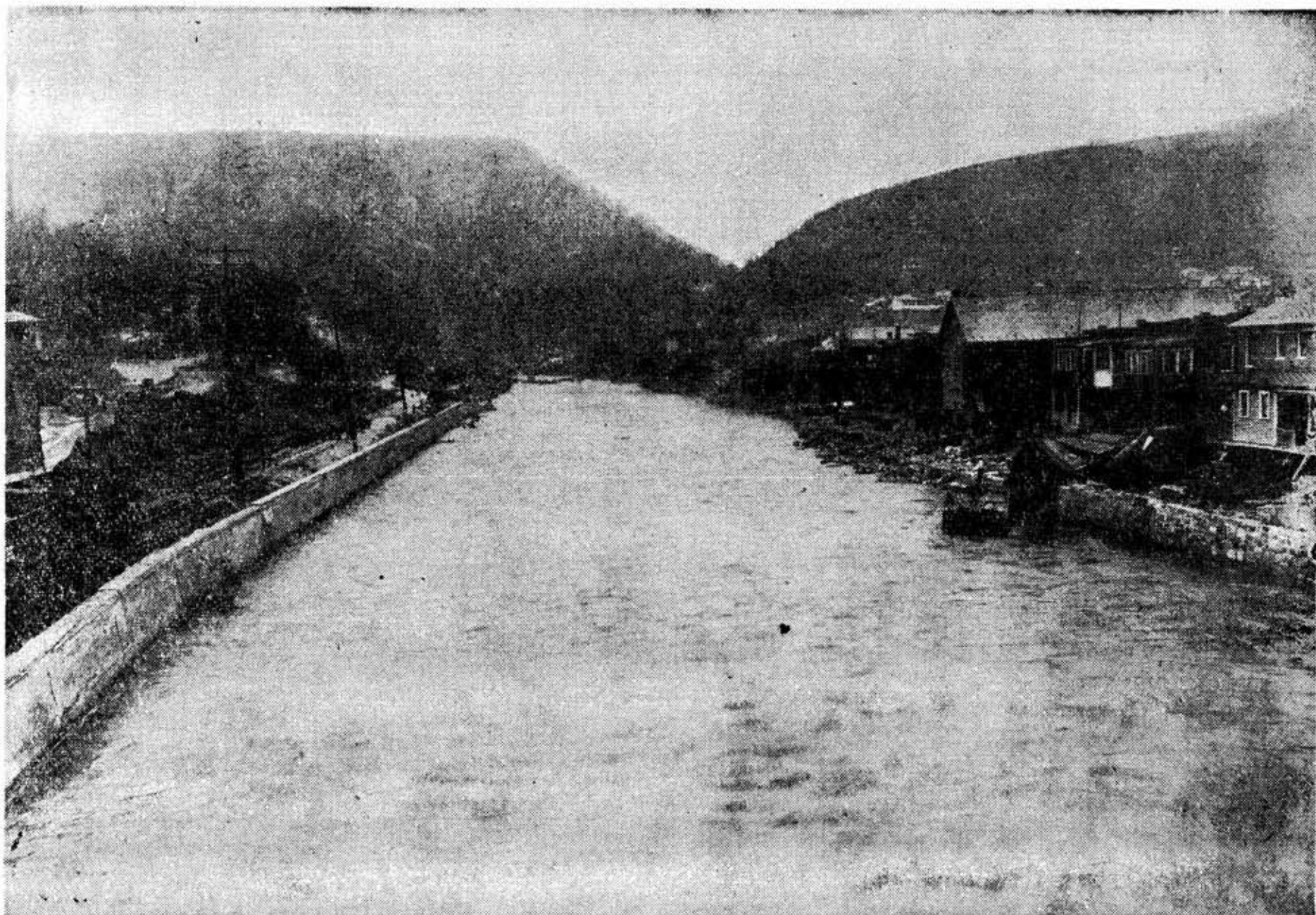
WILLS CREEK! NOTE THE SMASHED FREIGHT CAR ON THE RIGHT
