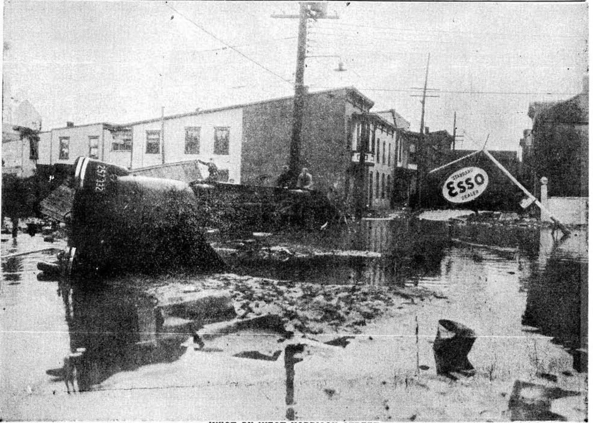
WEST ON WEST HARRISON STREET
