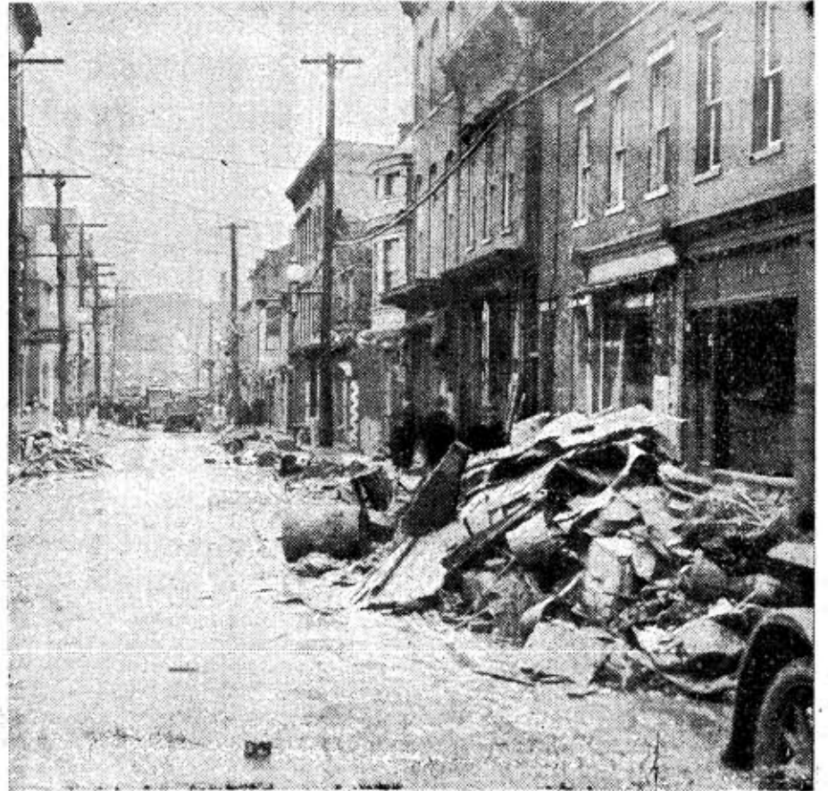
SOUTH CENTRE STREET, CUMBERLAND
