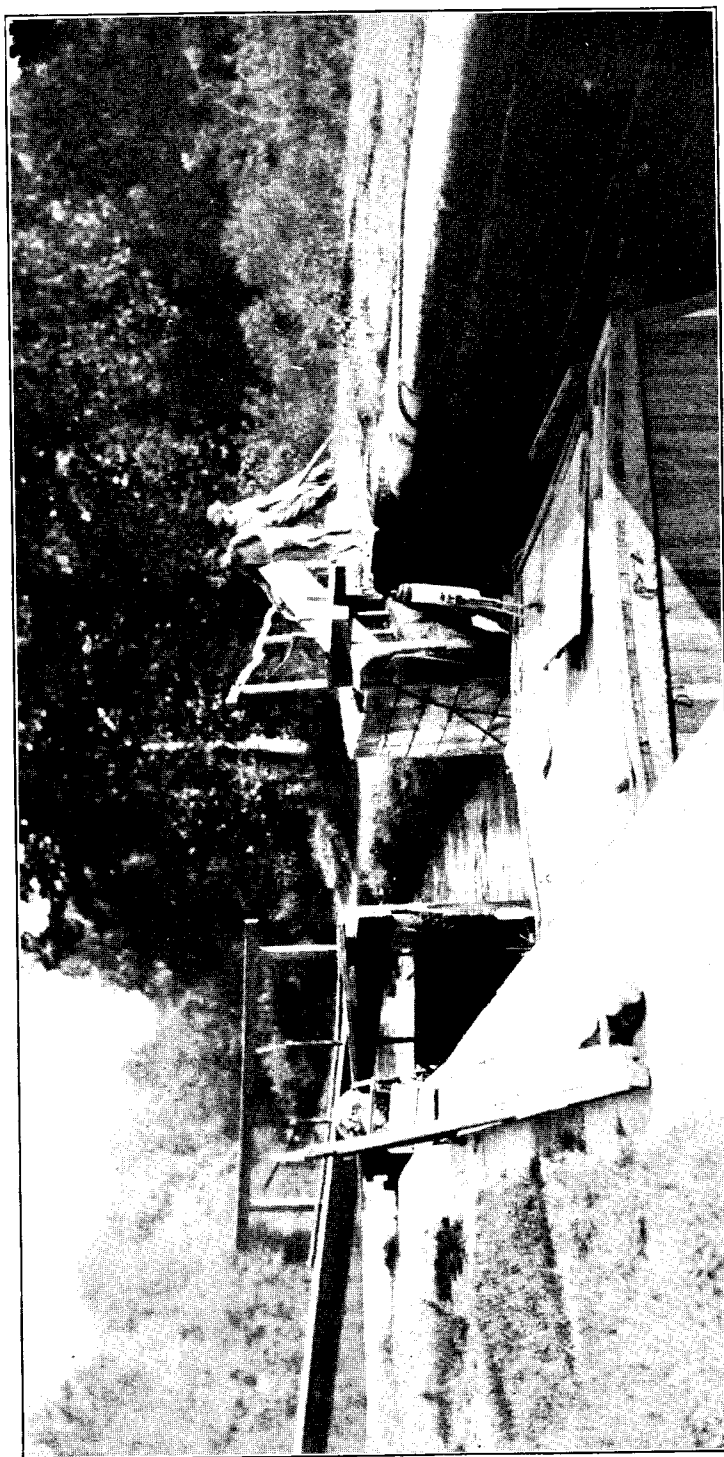
FIG. 3.—CAPTAIN AND TWO BOY HELPERS OPENING LOCK GATES. BOAT HAS BEEN LOWERED AND IS READY TO LEAVE LOCK.
