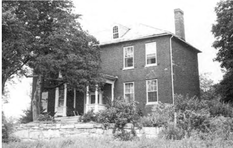
Fig. 3-013: Exterior of Ferry Hill Plantation House during Period Three (c1945), showing the south and west side of the west block. Note: storm windows, slate roof, snowboard at roof, loss of shutters, and masonry cracks between the windows of the first and second floors. (Collection J. Howard Beckenbaugh.)
