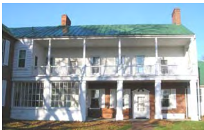
Fig. 3-007: South porch, 2004. The western enclosures on the first and second floors date to Period Two; the second story wood columns date to Period Five. (GWWO photo, 2004.)
