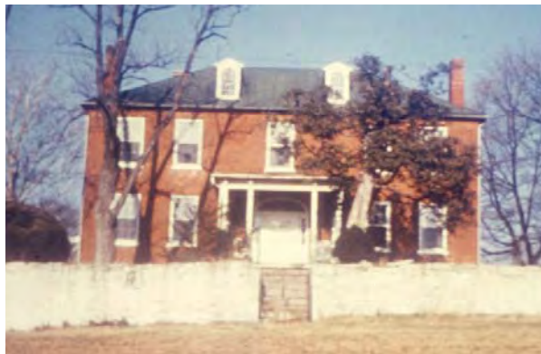
Fig. 3-014: Exterior of Ferry Hill Plantation House during Period Three (pre-1950), showing the west elevation of the west block. Note arrangement of front porch, slate roof, and loss of shutters. (C&O National Historical Park.)
