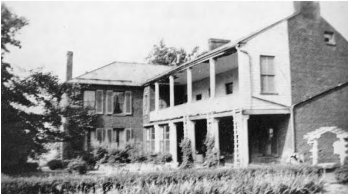
Fig. 3-011: Exterior of Ferry Hill Plantation House during Period Two (c1938), showing the east side of the west block and the east and south sides of the north leg, prior to the construction of the east addition. Note, east side downspouts, west block snowboard at roof, and lattice on columns. (Henry Kyd Douglas, / Rode with Stonewall , pg. 26.)
