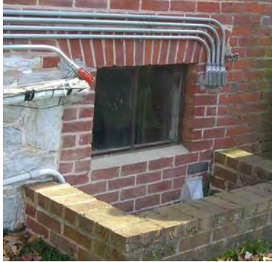
Fig. 3-015: Window 4A, where the change in brick shows evidence of an originally larger window. (GWWO photo, 2004.)
