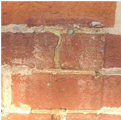
Fig. 3-006: Remnant of penciled masonry dating to Period One; west block, south elevation. (GWWO photo, 2004.)
