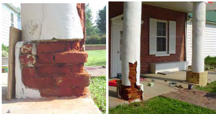
Fig. 3-023: South porch column bases, repair work undertaken in June 2004. Note paint remnants on several base bricks. This may indicate the columns were painted prior to the application of parging (Period Two). However these bricks are set in a grey mortar that does not match the adjacent mortar. (C&O National Historical Park.)
