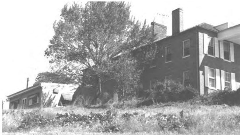
Fig. 3-020: Exterior of Ferry Hill Plantation House during Period Four (c1972), showing the north side and portions of the west side. Note, the northeast addition and two story porch exist. Shutters are missing from the north elevation. (C&O National Historical Park.)
