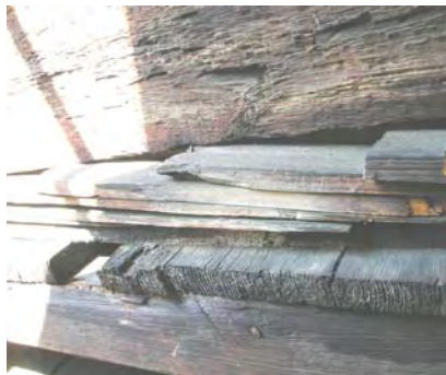
Fig. 3-004: Period One roof shingles sandwiched below the side framing member for the dormer. West roof, north dormer, north side, viewed from the attic. (GWWO photo, 2004.)
