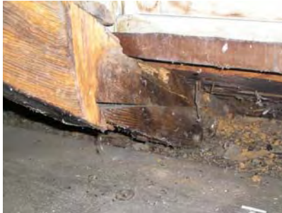
Fig. 5-014: Scarf joint failure condition at end of roof rafter. (GWWO photo, 2005.)
