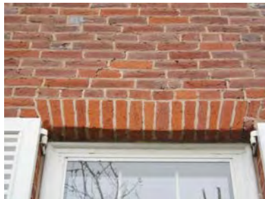
Fig. 5-006: Above: Brick jack arch over window 11, west block, north elevation. Cracks over the jack arch have caused the arch to sag in the center. Cracks actually shear bricks in several locations. At right: detail of cracks above the same window. (GWWO photo, 2005.)
