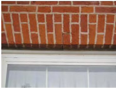
Fig. 5-007: Above: Jack arch over window 8, west block, south side, first floor of the west elevation. Joint surrounding keystone brick has cracked, and brick dropped about 1/8". (GWWO photo, 2005.)
