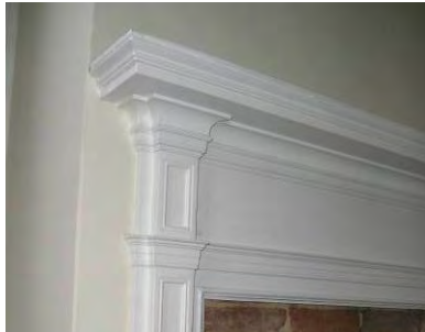
Fig. 4-083: Mantle shelf and upper pilaster (above), and overall fireplace (right). (GWWO photo, 2005.)
