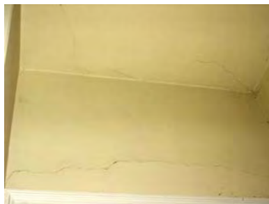
Fig. 5-017: Room 104, north wall and ceiling above window 12, showing plaster that has lost its key. (GWWO photo, 2005.)
