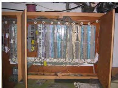
Fig. 4-270: Telephone punchdown blocks. (GWWO photo, 2005.)
