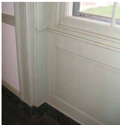
Fig. 4-064: Lower window inset panel. (GWWO photo, 2005.)
