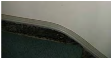
Fig. 4-074: Curved transition of base trim. (GWWO photo, 2005.)
