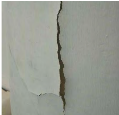
Fig. 4-107: Column paint peeling. (GWWO photo, 2005.)
