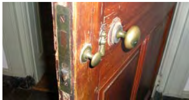
Fig. 4-063: Typical door hardware (Period One). (GWWO photo, 2005.)
