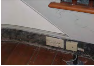
Fig. 4-260: Power and telephone outlets. (GWWO photo, 2005.)
