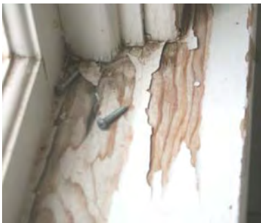
Fig. 5-025: Window 28, west side sill, showing peeling paint due to moisture exposure. (GWWO photo, 2005.)
