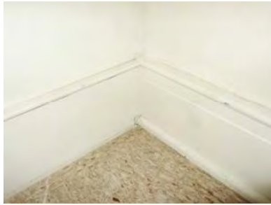
Fig. 4-211: Room 210, detail of Period One base (right) and base on chase wall (left). (GWWO photo, 2005.)
