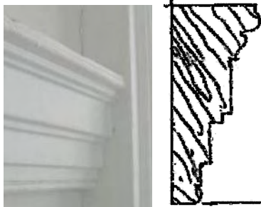
Fig. 4-092: Room 105 typical chair rail. GWWO photo, 2005; and GWWO section detail.
