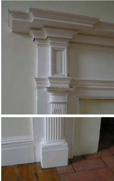
Fig. 4-154: Rm. 201 fireplace (right). Detail of mantel shelf and upper pilaster (upper left); detail of lower pilaster (lower left). (GWWO photo, 2005.)
