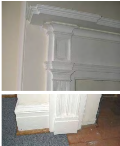
Fig. 4-095: Mantle shelf and upper pilaster (top left); Fireplace overview (right); Lower pilaster and hearth (bottom left). (GWWO photo, 2005.)
