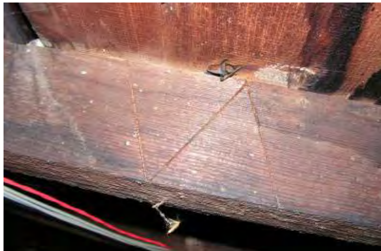
Fig. 4-227: Examples of marriage marks on the rafters (above and right). Marriage mark that appears to be a reverse "N" (right). (GWWO photo, 2005.)
