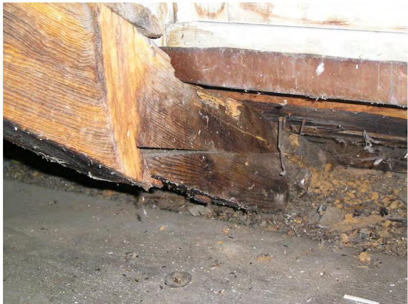
Fig. 4-239: Scarf joint at end of roof rafter. (GWWO photo, 2005.)
