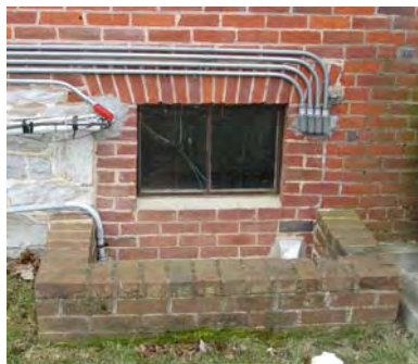
Fig. 4-033: Two views of the brick areaway and basement window. North elevation, west block. The foundation material changes from brick to local limestone at the east side of this opening. (GWWO photo, 2005.)
