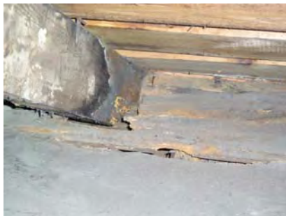
Fig. 5-015: Roof rafter and deck deterioration caused by water infiltration at the eave line. (GWWO photo, 2005.)
