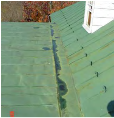
Fig. 5-001: View of joint between west block and west porch, looking north. Ponding of water is evident two days after last rain. (GWWO photo, 2005.)
