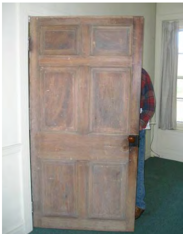
Fig. 5-024: Door 28, between Rooms 206 and 208, showing wear from exterior exposure. (GWWO photo, 2005.)
