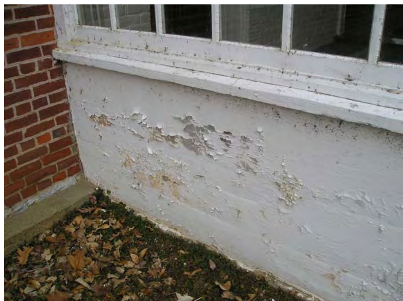
Fig. 5-011: Examples of paint failure. Top: window 29, east elevation, west block, first floor. Paint is exfoliating from sill and portions of window casing. Bottom: painted concrete base below glazing of Entry 106, south elevation, north leg. (GWWO photo, 2005.)
