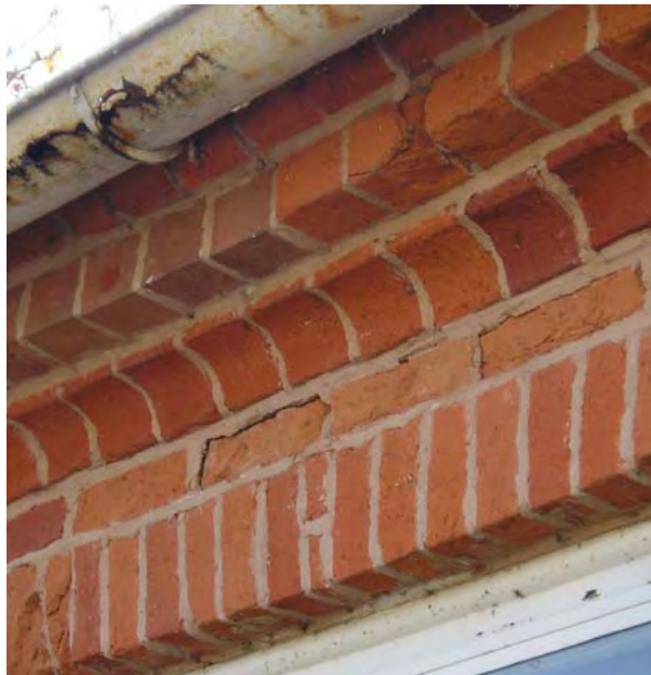
Fig. 5-007: Above: Jack arch over window 8, west block, south side, first floor of the west elevation. Joint surrounding keystone brick has cracked, and brick dropped about 1/8". (GWWO photo, 2005.)
