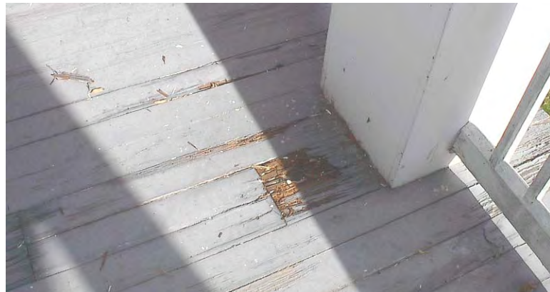
Fig. 4-234: At right: water damage at porch deck, space 207. (GWWO photo, 2005.)
