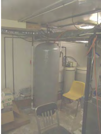
Fig. 4-253: Well Water Treatment Equipment. (GWWO photo, 2005.)
