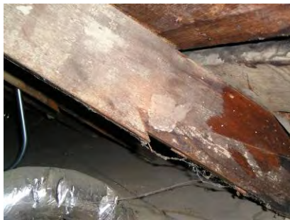
Fig. 4-239: Scarf joint at end of roof rafter. (GWWO photo, 2005.)
