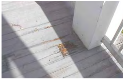
Fig. 5-012: View of deteriorated floor decking at south porch. Water has rotted the material. (GWWO photo, 2005.)
