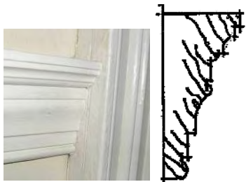
Fig. 4-093: Room 105 chair rail found on the northwest wall. (GWWO photo, 2005) and section detail.
