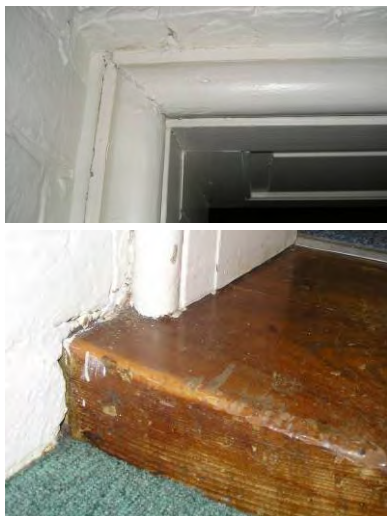
Fig. 4-109: Door 12 details, bullnose door trim (upper), and wood threshold (lower). (GWWO photo, 2005.)
