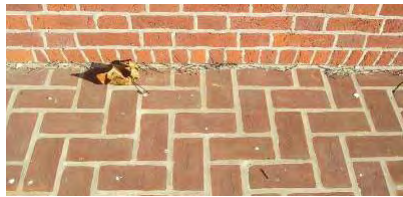
Fig. 4-019: Detail of west elevation masonry at porch floor. The top of a jack arch for basement window 02 is visible above the porch deck. (GWWO photo, 2004.)
