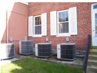
Fig. 4-244: Air Cooled Condensing Units. (GWWO photo, 2005.)
