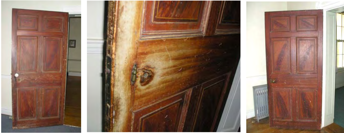
Fig. 5-023: Left to right: A) Door 8 to Room 104, has scratching on the hall side; B) Door 9 between Rooms 104 and 105 has excessive wear at the zone of the hardware; and C) Door 28 to Room 201 has scratches on the hall side. (GWWO photo, 2005.)
