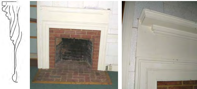
Fig. 4-204: Profile of mantle shelf (above); profile of wood surround (right); overall fireplace (right center); detail of mantle shelf and surround (far right). (GWWO photo, 2005.)
