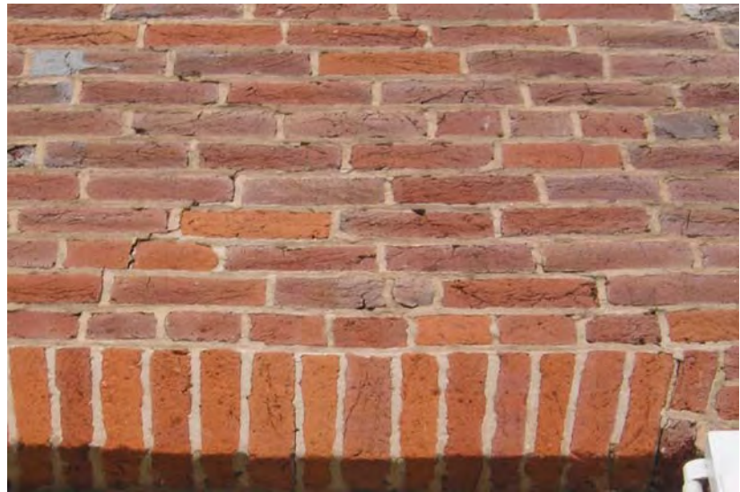
Fig. 5-006: Above: Brick jack arch over window 11, west block, north elevation. Cracks over the jack arch have caused the arch to sag in the center. Cracks actually shear bricks in several locations. At right: detail of cracks above the same window. (GWWO photo, 2005.)
