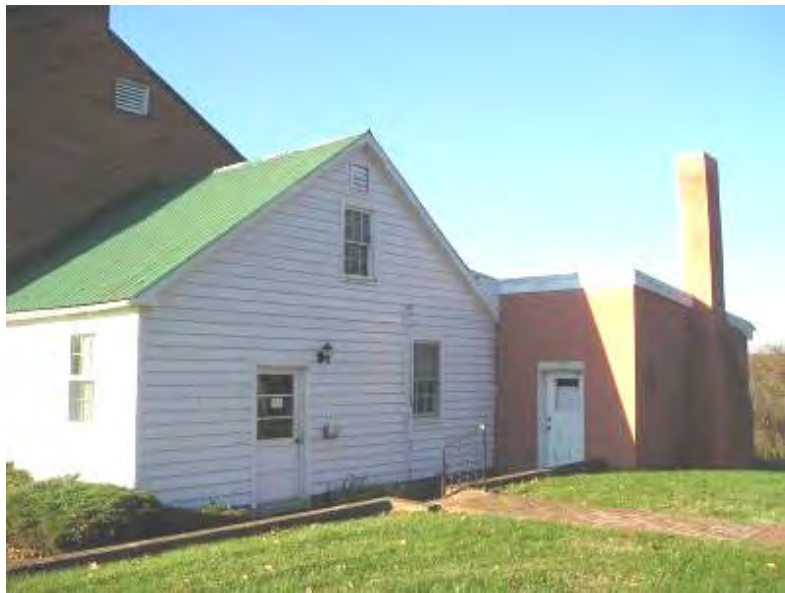
Fig. 4-035: South and east elevations of the east addition. To the right (north) of this addition, portions of the subsequent northeast (cmu) bar addition are visible. (right). Detail of double-ribbed metal roofing (above). (GWWO photo, 2005.)
