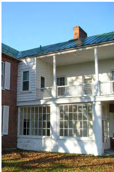
Fig. 4-027: North Leg, South Elevation, detail at west side showing glazed first floor Entry 106 and enclosed second floor Bath 203. (GWWO photo, 2004.)
