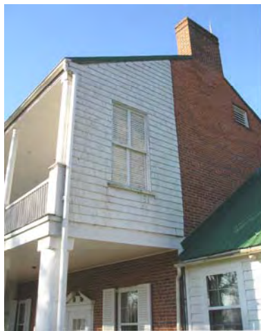
Fig. 4-031: Second floor south porch, east elevation of east wing wall, showing wood siding (Period One), double-hung louver (Period One), and downspout (Period Five) running straight down beside both second and first floor columns. (GWWO photo, 2005.)
