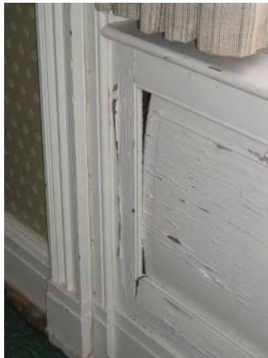
Fig. 4-184: Damage at lower window panel, window 39. (GWWO photo, 2005.)
