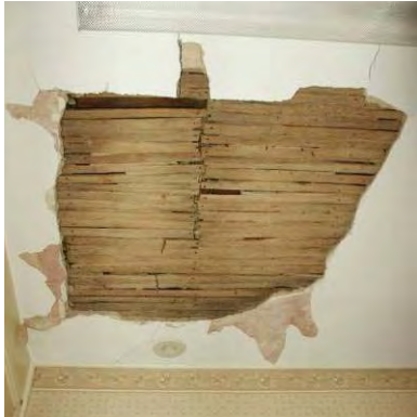
Fig. 5-018: Room 107, ceiling above window 26, showing area of missing plaster. (GWWO photo, 2005.)
