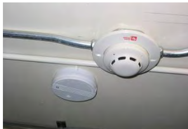
Fig. 4-266: Smoke detectors. GWWO photo, 2005.
