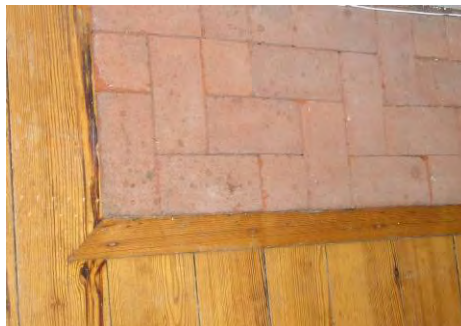
Fig. 4-156: Fireplace pilaster section: upper portion (above left) and lower portion (above right). Mitered border at front face of hearth (right). (GWWO photo, 2005.)
