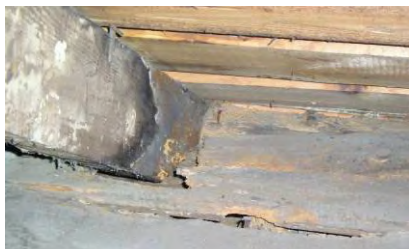
Fig. 4-238: Roof rafter and deck deterioration caused by water infiltration at the eave line. (GWWO photo, 2005.)
