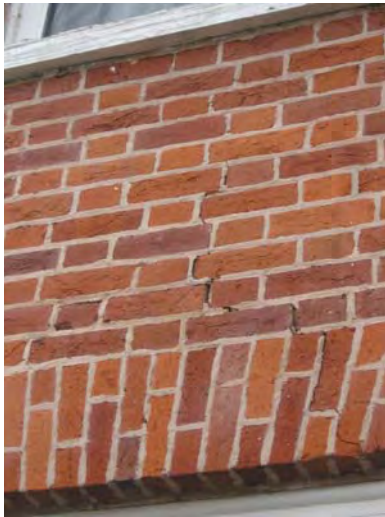
Fig. 5-005: Cracks in masonry over window 10, west block, west elevation. (GWWO photo, 2005.)
