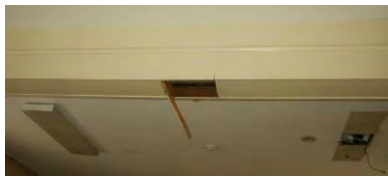
Fig. 4-116: Eastern ceiling beam, showing portion opened for investigation. (GWWO photo, 2005.)
