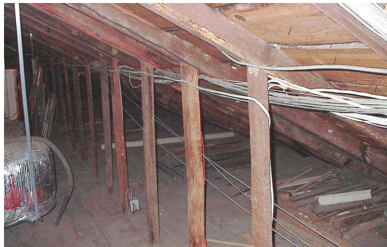
Fig. 4-236: Interior post supports at roof rafters, typical. (GWWO photo, 2005.)
