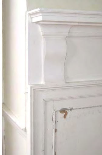
Fig. 4-171: Chair rail on north face of chimney projection, which is unevenly installed and has a crudely truncated end (above); detail of mantle shelf and surround (center); overall fireplace (right). (GWWO photo, 2005.)
