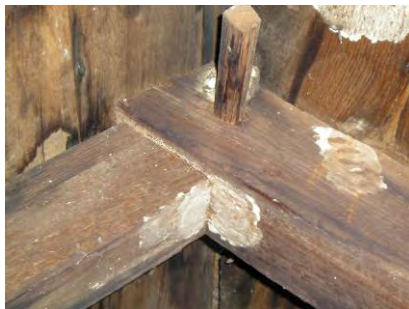
Fig. 4-235: Hand hewn wooden nail at joint between roof rafters. (GWWO photo, 2005.)
