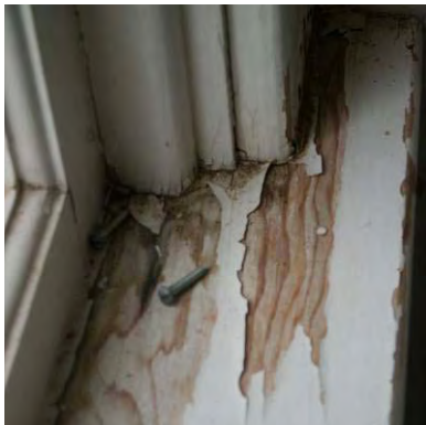
Fig. 4-113: Windows 27 and 28 sill and trim paint peeling. (GWWO photo, 2005.)
