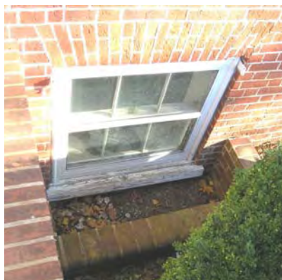
Fig. 4-017: Basement three-over-three window, with shutter hardware, and surrounding window well. (GWWO photo, 2005.)
