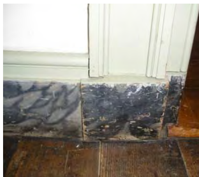
Fig. 4-039: Example of typical faux-marble base. (GWWO photo, 2004.)
