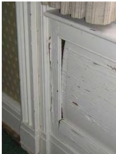
Fig. 5-020: Room 205, north wall, under window 39, showing warped wood panel probably due to moisture infiltration. (GWWO photo, 2005.)
