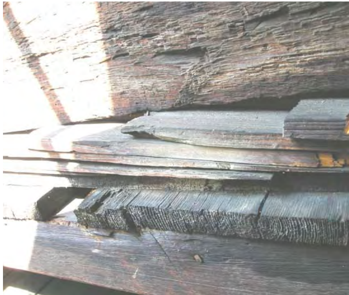
Fig. 4-228: Exposed lath behind the finished plaster on the two walls that flank the steps. (GWWO photo, 2005.)
