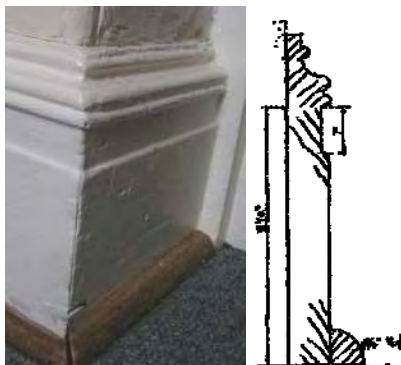
Fig. 4-094: Room 105 base. (GWWO photo, 2005), and section detail.
