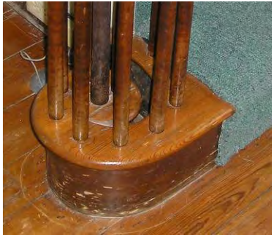
Fig. 4-077: Lateral scroll terminus at lowest stair tread. (GWWO photo, 2005.)
