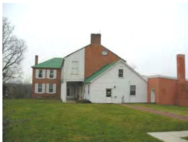
Fig. 4-036: East Elevation showing east addition. To the left (south) of the addition, the east elevation of the north leg and the east elevation of the west block are both visible. To the right (north) of the addition, a segment of the later northeast (cmu) addition is visible. (GWWO photo, 2005.)
