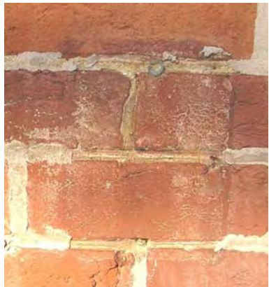
Fig. 4-022: Main Block, south elevation, detail at remnant of penciling. (GWWO photo, 2005.)
