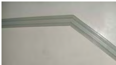
Fig. 4-073: Mitered transition of chair rail. (GWWO photo, 2005.)
