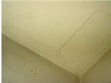
Fig. 5-016: Room 101, southwest corner at ceiling, showing sagging plaster that has lost its key to the lath above. (GWWO photo, 2005.)
