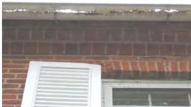
Fig. 5-004: Gutter over window 51, west block, east elevation. Daylight can be seen through the holes of the gutters. (GWWO photo, 2005.)
