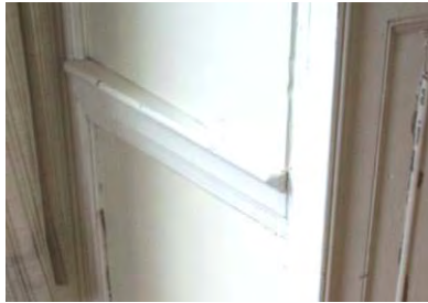
Fig. 4-171: Chair rail on north face of chimney projection, which is unevenly installed and has a crudely truncated end (above); detail of mantle shelf and surround (center); overall fireplace (right). (GWWO photo, 2005.)
