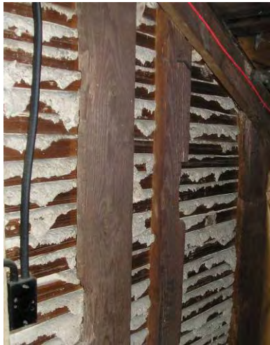
Fig. 4-228: Exposed lath behind the finished plaster on the two walls that flank the steps. (GWWO photo, 2005.)
