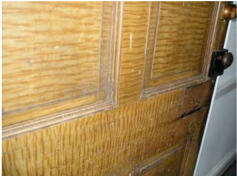
Fig. 4-102: Room 105, door 10, showing detail of bird's eye tiger maple painted graining. The reason for the change in graining style from the rest of the house, is unknown. (GWWO photo, 2005.)
