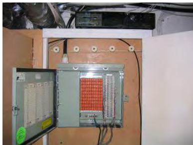
Fig. 4-269: Telephone protection blocks. (GWWO photo, 2005.)
