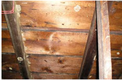
Fig. 4-237: Roof rafter and deck, showing "skipped" sheathing. (GWWO photo, 2005.)
