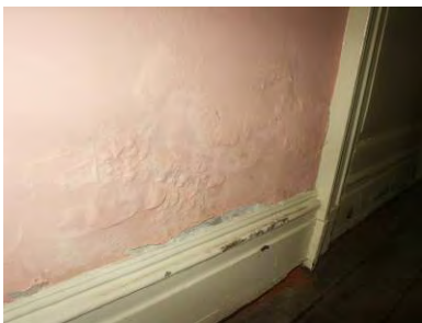
Fig. 5-019: Room 107, south wall, showing spalling plaster due to moisture damage. (GWWO photo, 2005.)
