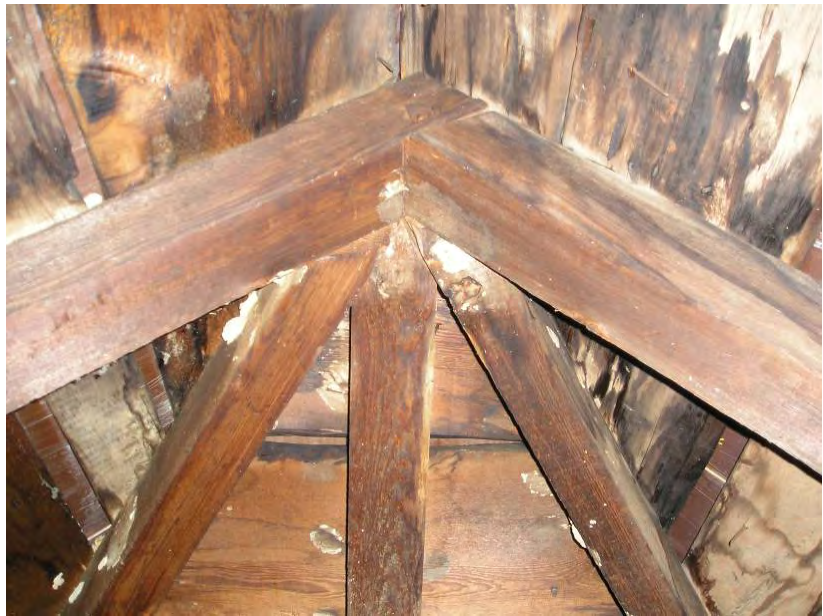
Fig. 4-226: Detail drawings of the roof ridge section and construction connections (above); hip peak with mortise and tenon joints (right). (GWWO photo, 2005.)
