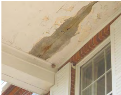
Fig. 5-013: Two views of deteriorated plaster ceiling at west porch. Water damage has been caused by failure in the roof. (GWWO photo, 2005.)
