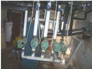
Fig. 4-247: Boiler and 5 Zone Circulators. (GWWO photo, 2005.)
