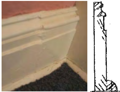
Fig. 4-121: Room 107 base, showing transition from Period Four base to Period One base, north of the fireplace (left). GWWO photo, 2005. Period One base profile (right).
