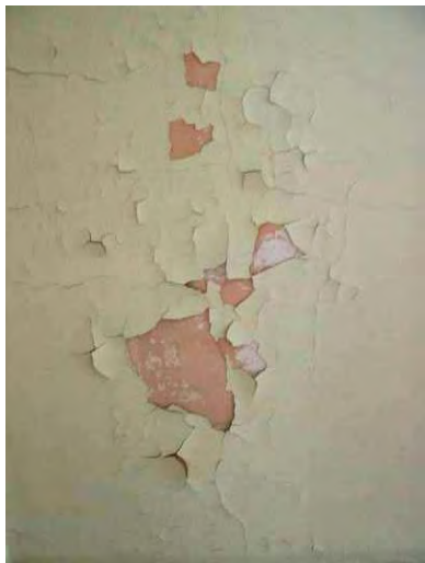
Fig. 5-028: Room 204, large patch of paint peeling. (GWWO photo, 2005.)
