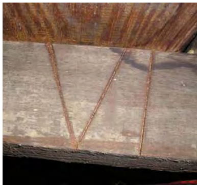
Fig. 4-227: Examples of marriage marks on the rafters (above and right). Marriage mark that appears to be a reverse "N" (right). (GWWO photo, 2005.)
