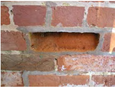
Fig. 5-009: Masonry stretcher course immediately below first header course, south elevation, north leg, under south porch, below window 26. One brick has lost the entirety of its surface, and over half of its body, to spalling. (GWWO photo, 2005.)
