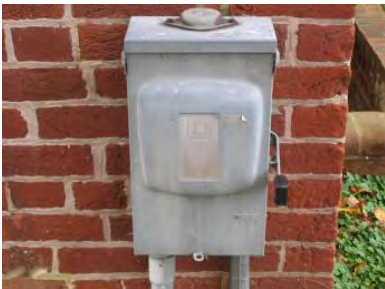
Fig. 4-262. Unused service disconnect. (GWWO photo, 2005.).
