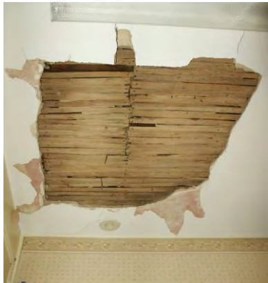
Fig. 4-115: Exposed lath to the west of the western beam on the south portion of the ceiling. (GWWO photo, 2005.)
