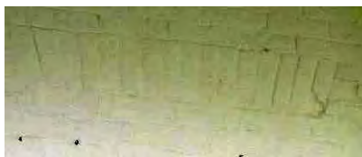
Fig. 4-106: Remaining jack arch shows evidence of the previous opening. (GWWO photo, 2005.)
