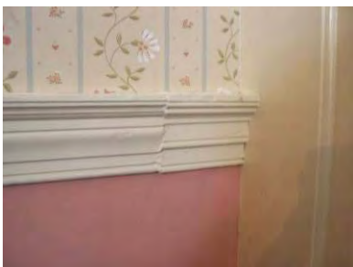
Fig. 4-120: Transition from Period Four replacement trim to Period One trim north of the fireplace (above). South wall, below chair rail which shows peeling, cracking and exfoliation (center and right). (GWWO photo, 2005.)
