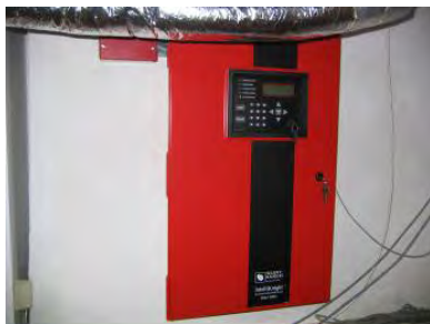
Fig. 4-265: Fire alarm panel. (GWWO photo, 2005.)
