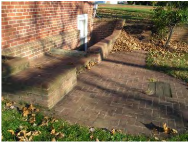
Fig. 4-021: Main Block, south elevation, showing brick areaway and water table (Period Four). (GWWO photo, 2004.)
