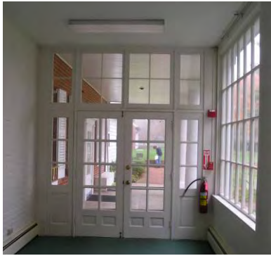
Fig. 4-110: Door 13, French doors with transom and side lites. (GWWO photo, 2005.)
