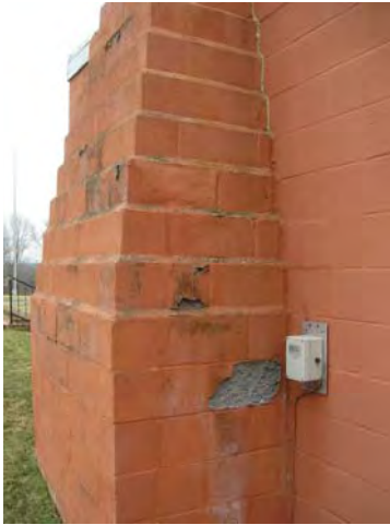
Fig. 5-010: CMU masonry at east elevation of northeast addition . The corbelled block surrounds the fire chamber of the fireplace located on the inside. Block surfaces have exfoliated and spalled, probably due to their inability to withstand the heat generated in the fireplace. (GWWO photo, 2005.)
