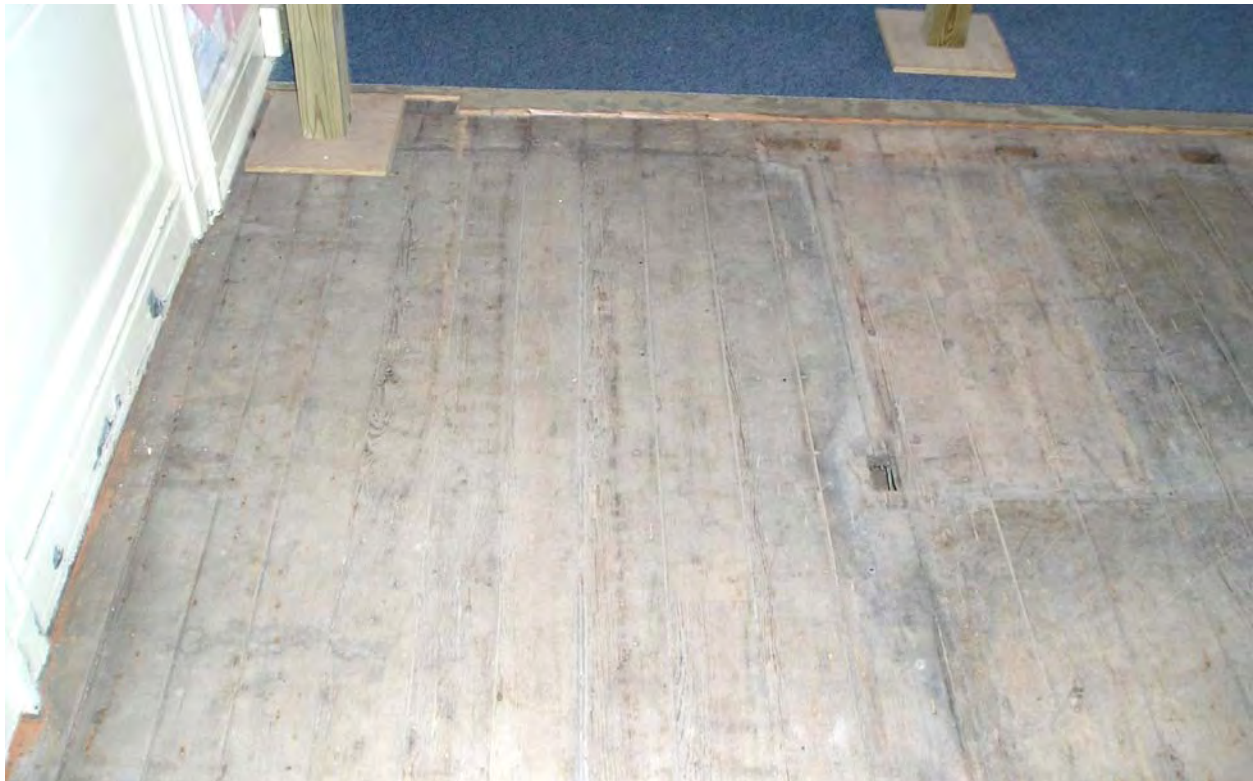
Fig. C-014. Room 107, south end of the stair-pantry area, looking west. The central stud hole marks the transition from pantry portal (east of the hole) to first riser of the stairs (west of the hole). The clear line of the first riser is visible, as is the casing marks for door to the dining room. (GWWO photo, 2005)
