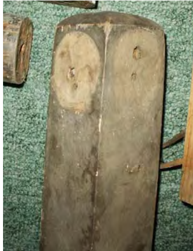
Fig. C-005. View of Newel post 3, showing ghosts of railings and base condition. (GWWO photo, 2005)
