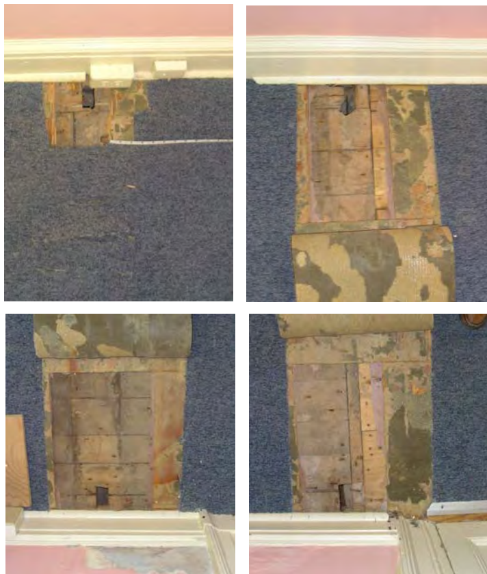
Fig. C-013. Selective demolition at first floor dining room 107, showing remnants of the wall conditions of the pantry. Images clockwise from upper left show northwest, northeast, southeast and southwest corners. The west wall of the pantry was located approximately 35" east of the north door in the original dining room. Ghost marks and stud holes from the original walls are evident. The threshold mark lending to the dining room is evident in the southeast image, beginning approximately 6-3/4" off the south wall. (GWWO photo, 2005)
