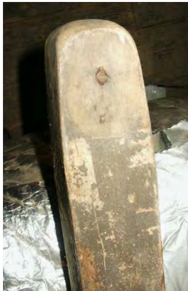
Fig. C-006. View of Newel post 4, showing ghost of railing and base condition. (GWWO photo, 2005)
