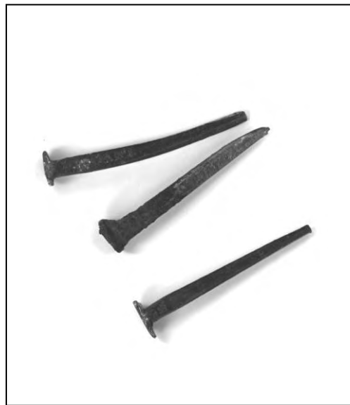
Fig. C-020. Lath nails, details showing "irregular heads which vary in size and shape." As noted by Nelson, the nails generally have "rather distinct rounded shank (under head)." (GWWO photo, 2005)
