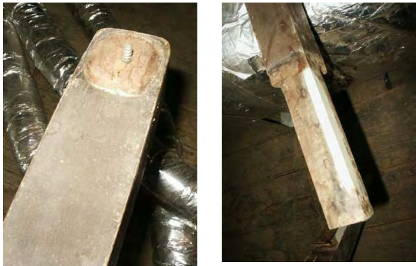
Fig. C-004. View of Newel post 2, showing ghost of railing and base condition. (GWWO photo, 2005)
