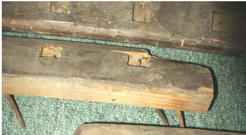
Fig. C-009. (left) View of the base components of the second floor rail system. Upper piece is the north Base D showing bull nosed edge. Lower piece is east base C, seen from its side that butted the adjacent flooring. (GWWO photo, 2005)
