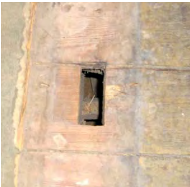
Fig. C-016. Stud hole at west wall of pantry. The “ghost” of the full 4” by 4” stud is clearly visible. The 1-1/2” tongue extended down below the floor. The floor boards were cut out after their installation. (GWWO photo, 2005)
