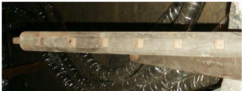
Fig. C-007. View of the Railing A, looking toward the end with the projecting tenon that inserted into the wall. (GWWO photo, 2005)
