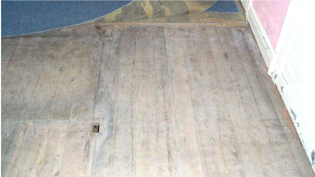
Fig. C-015. Room 107, south end of the stair-pantry area, looking east. Two studs flank the ends of the threshold that defined the entry into the pantry zone of the floor plan. (GWWO photo, 2005)
