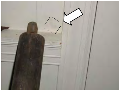
Fig. C-012. View of the west end of rail D, set adjacent to patch mark (indicated by white arrow and the dotted lines) where it was originally positioned in the wall. View is at south casing of attic door. (GWWO photo, 2005)
