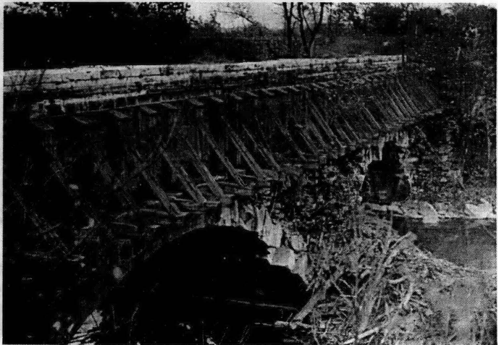
Figure 18. Berm side of the Conococheague Aqueduct with wood parapet, circa 1939. (Chesapeake and Ohio Canal National Historical Park Photo Library)
