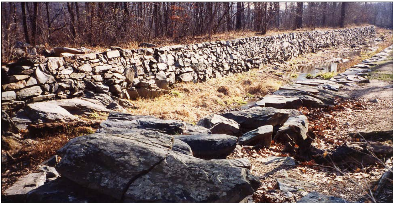
Reconstructed walls of the Great Falls canal. (D. Guzy)
