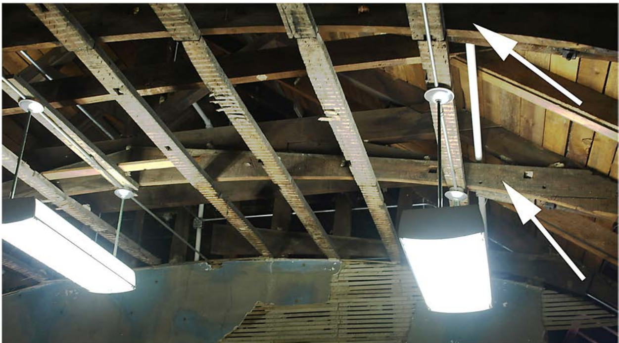
Gondola sideboards carved into curved joists. The stingers nailed below the joists were cut from gondola ribs. (D. Guzy)
