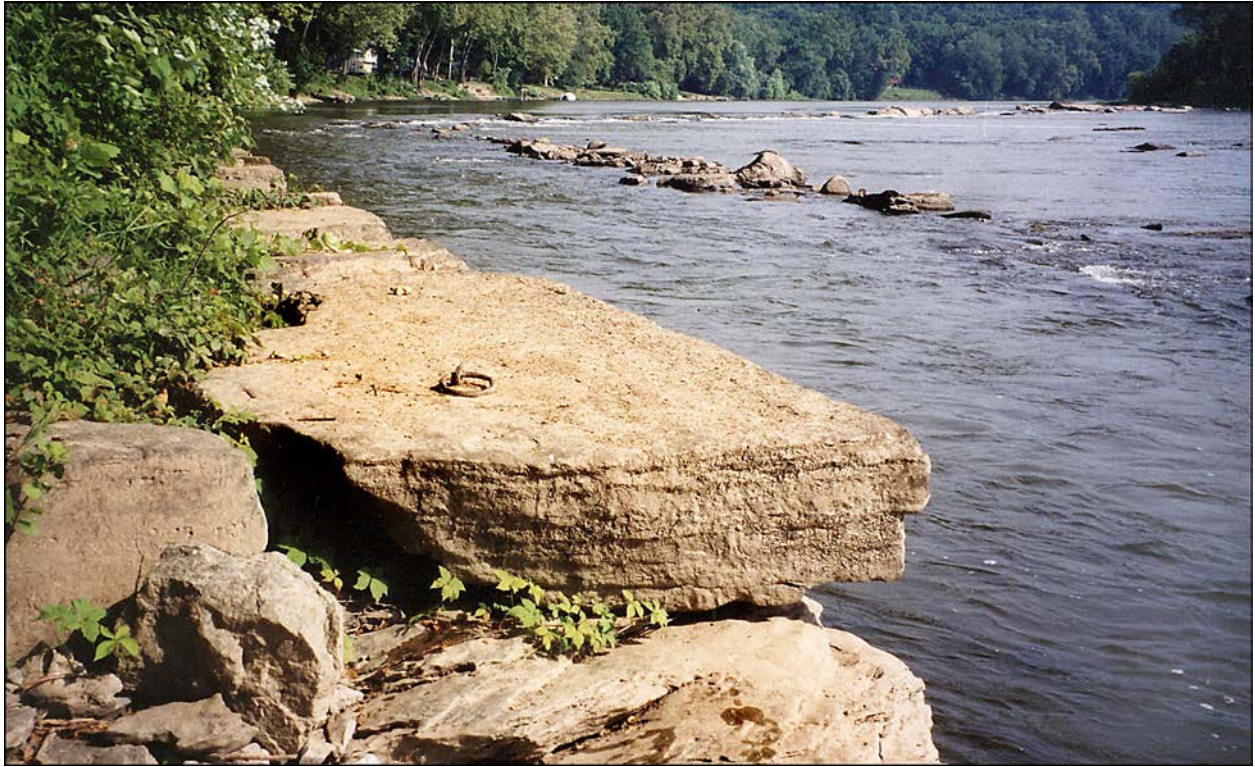
House Falls sluice, looking upstream. Note rock ledge in background, parallel wall and weir, and ring on the wall. (D. Guzy)
