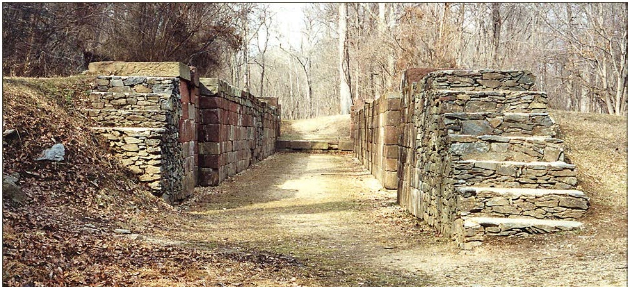
Lock seats for the Potomac Company's Lock No. 1 at Great Falls. (D. Guzy)
